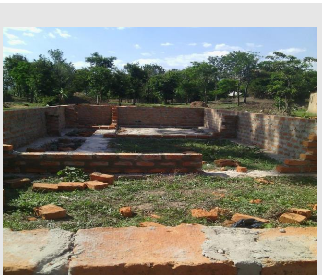
Photo 2: Construction of the new ICT lab at Nyanza primary school
